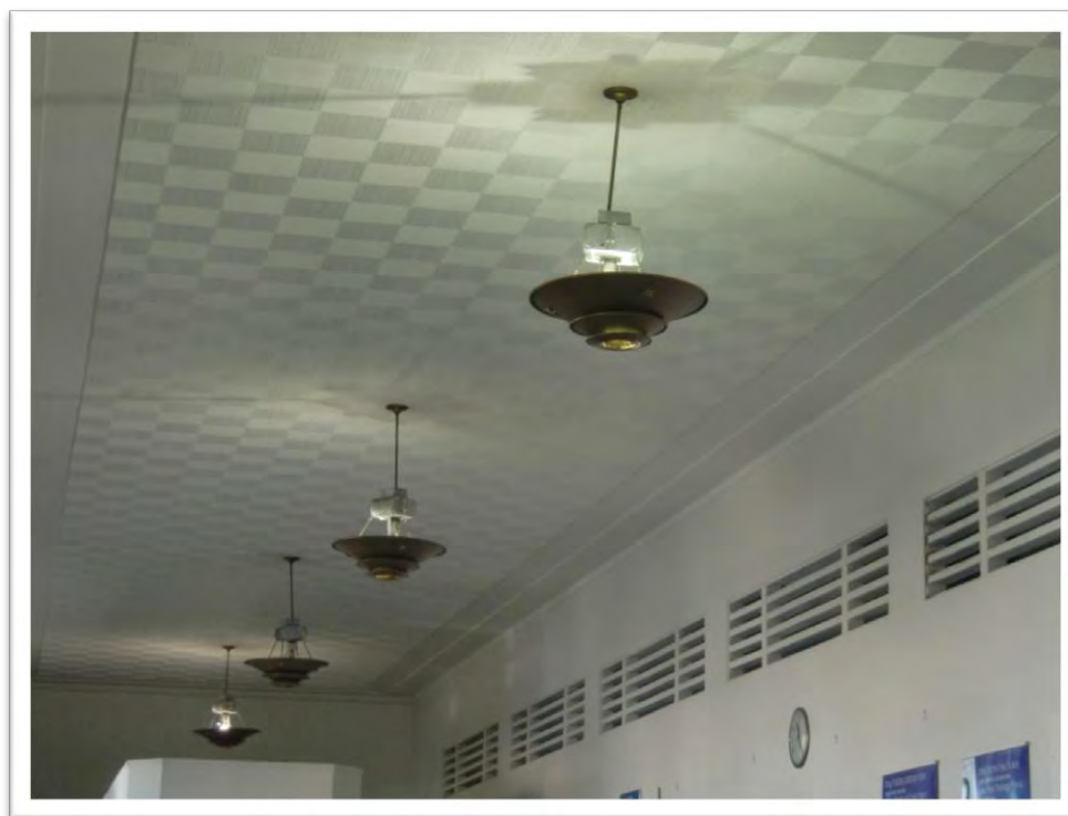
Photograph 10: Original hanging light fixtures in lobby
