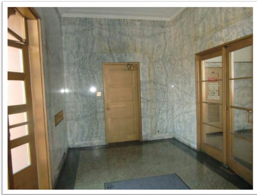
Photograph 11: Vestibule with marble walls and brass trim
