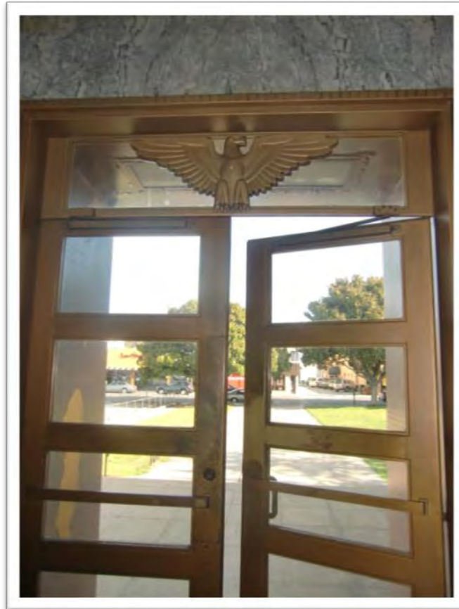
Photograph 9: Interior of entry door with eagle relief
