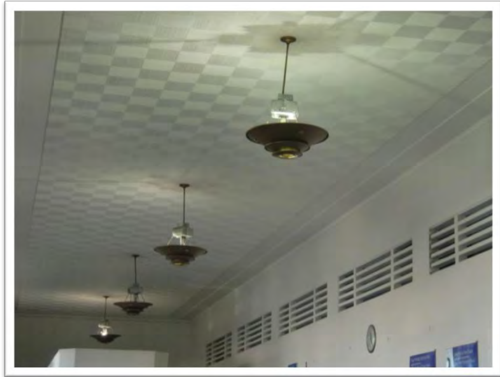
Photograph 7: Original hanging light fixtures in lobby
