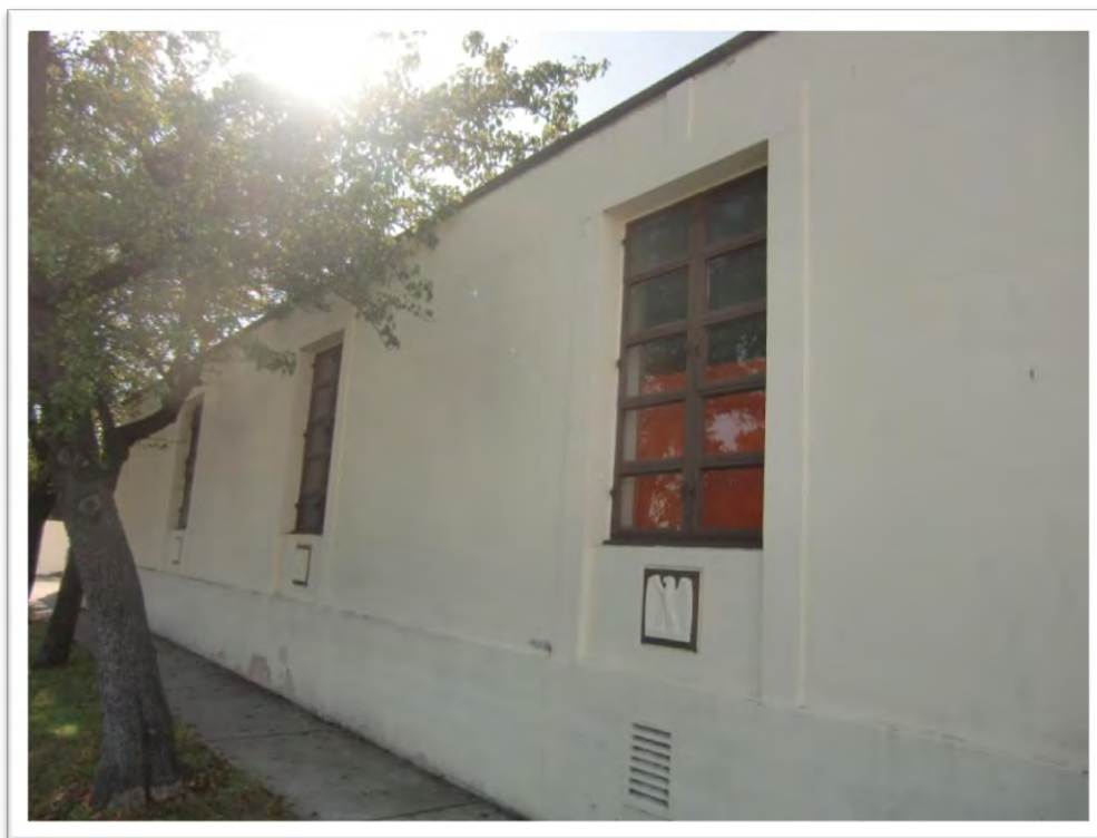
Photograph 7. Burlingame Post Office, window detail
