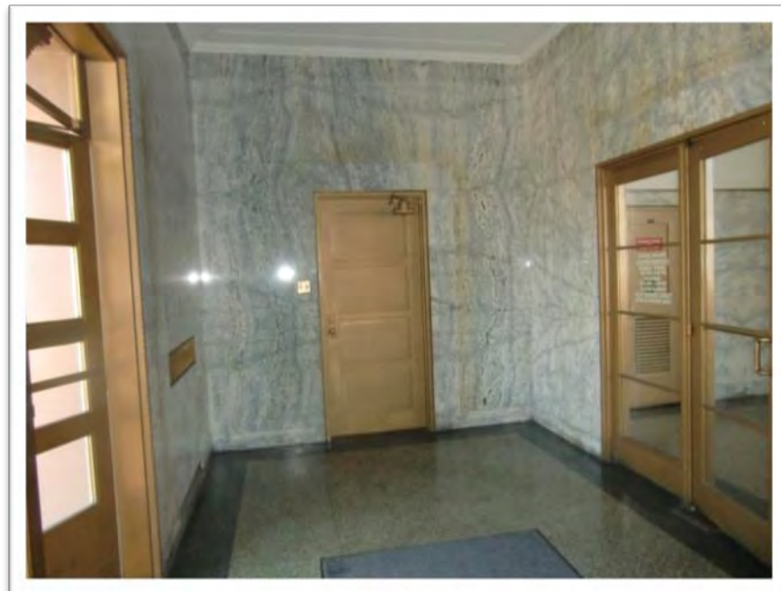
Photograph 8: Vestibule with marble walls and brass trim
