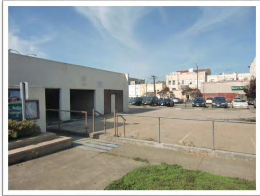
Photograph 14: Detached garage addition
