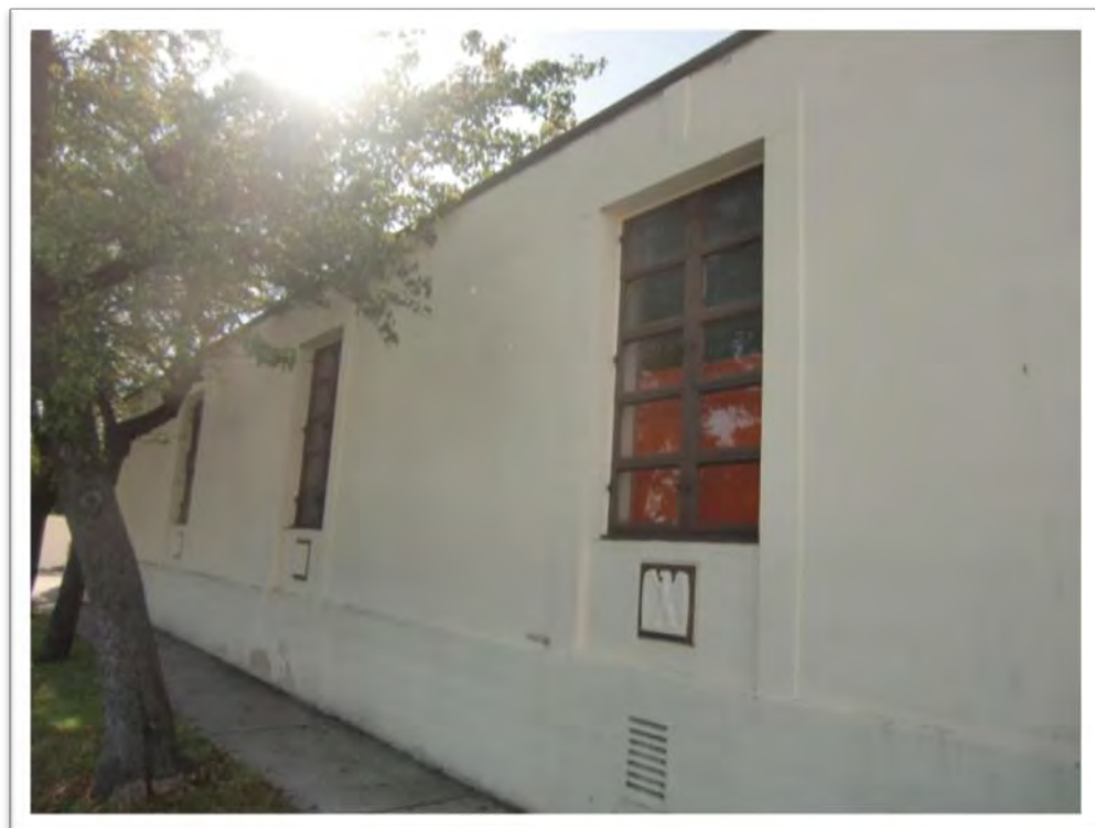
Photograph 4. Burlingame Post Office, window detail
