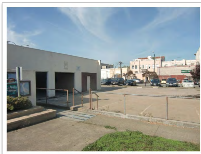
Photograph 17: Detached garage addition
