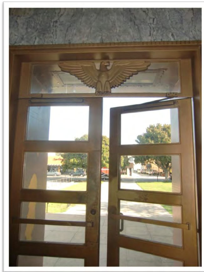
Photograph 12: Interior of entry door with eagle relief
