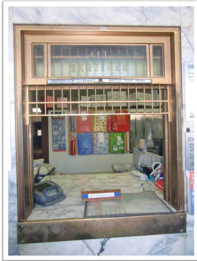
Photograph 11: Original service window
